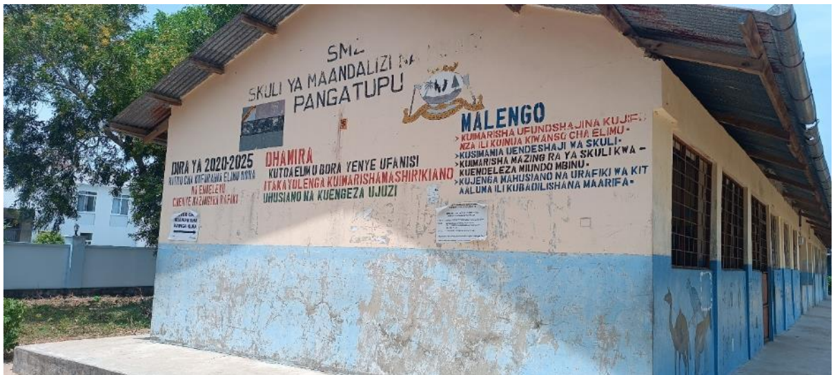
Figure 4-10: Pangatupu Primary School Source: Field data
